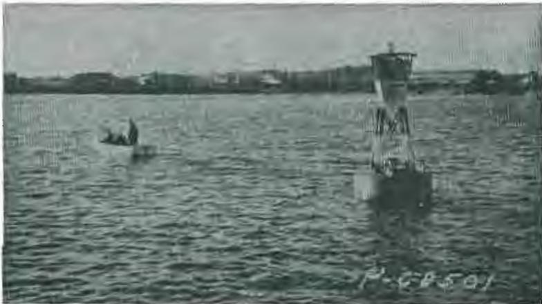
Nuclear-powered light buoys were put in place, this one off Baltimore. These and the "deep sea weather station" used strontium-90 as fuel.
